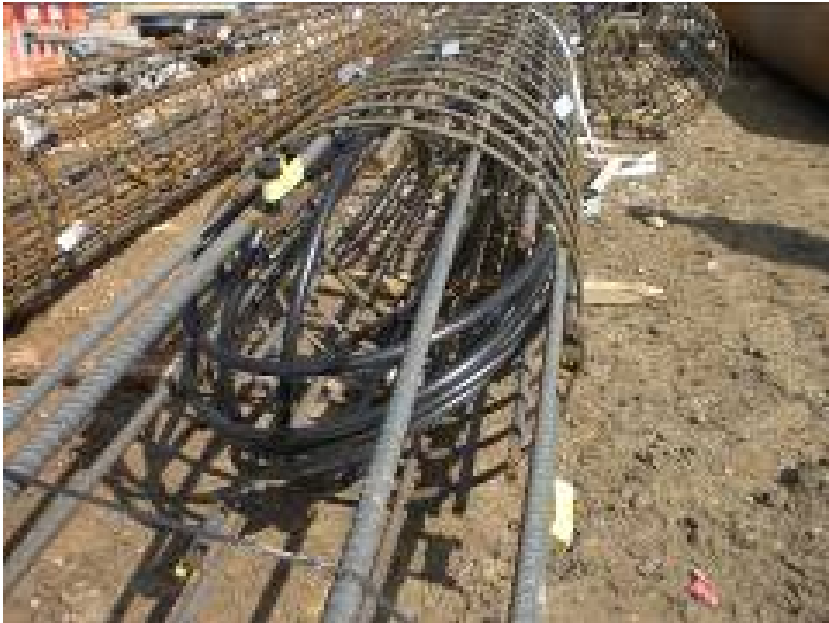
Geothermal Piles at One New Change, Arup (2009)
